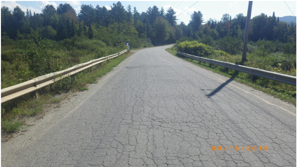
Looking South Over Bridge
