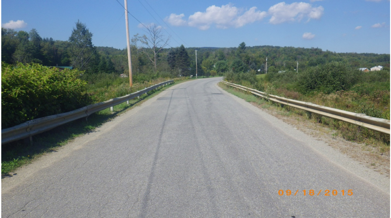
Looking North Over Bridge
