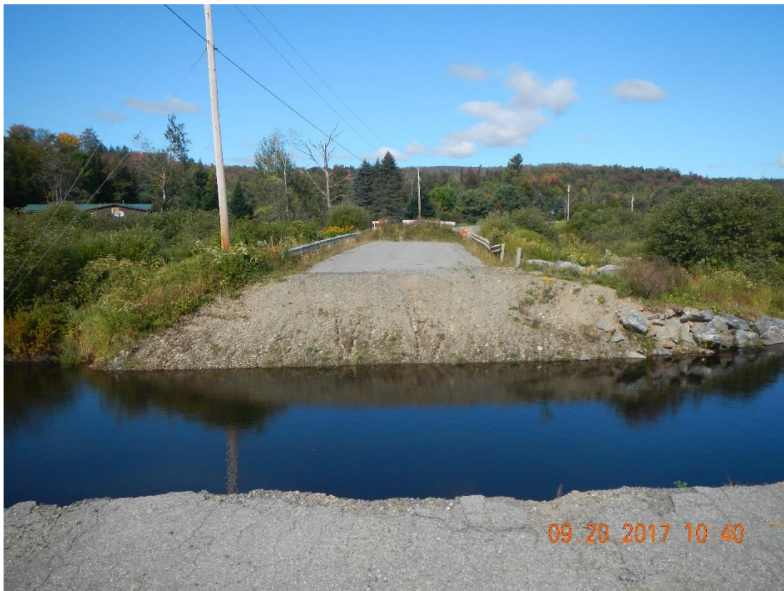
Figure 2: Looking northwest across river; visible are overhead wires running parallel to roadway and large stone fill on river bank.
